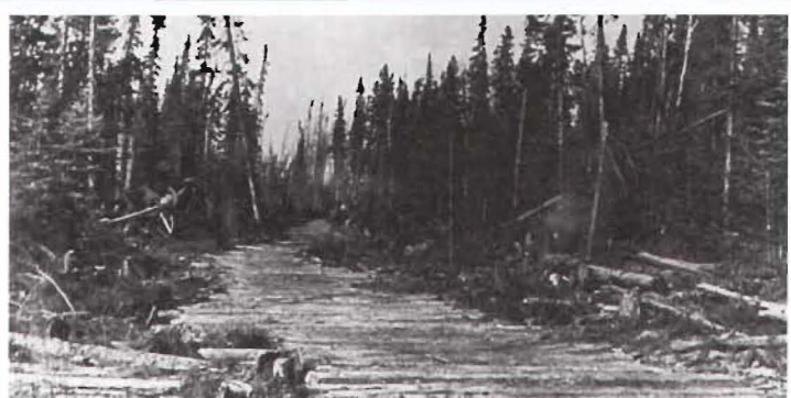
People travelling on Upper Canada's roads in the 1800s often encountered sections of deep mud. One of the solutions was called the "corduroy road," shown here. Trees were cut and placed tightly together over these wet areas so wagons and sleds could cross; however, they were very uncomfortable for travellers.
